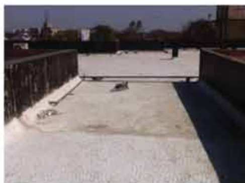
New cooling technologies used in Ahmedabad to combat the UHI effect: china mosaic roof tiles
