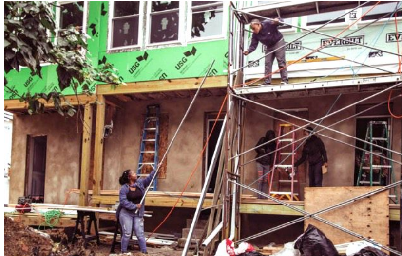
Retrofit & renovation – Baltimore
