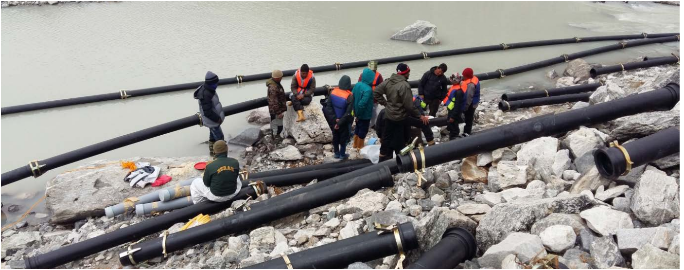
Installation of siphon system
