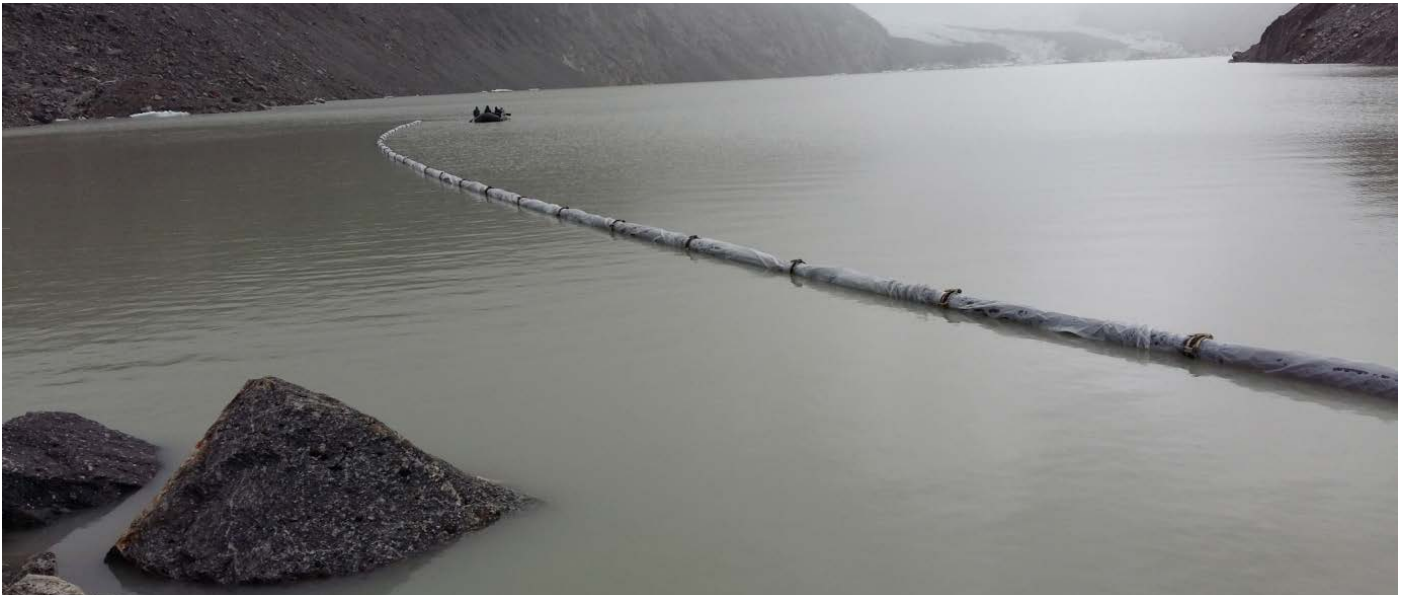
Siphon System after installation
